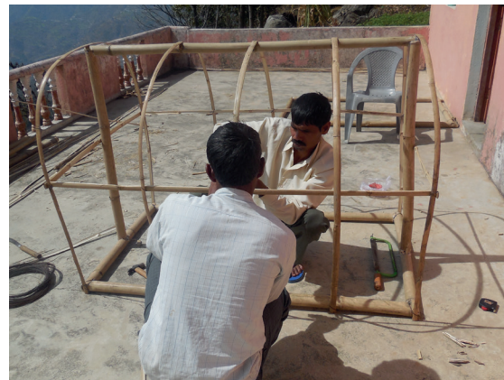
Solar poly tunnel dryer; drying vegetables; and construction of the top part from bamboo.
