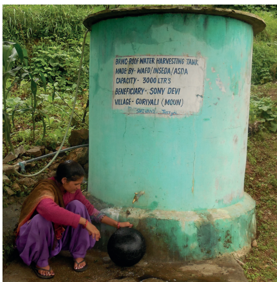
Bamboo reinforced rain water tank in India built by INSEDA.
