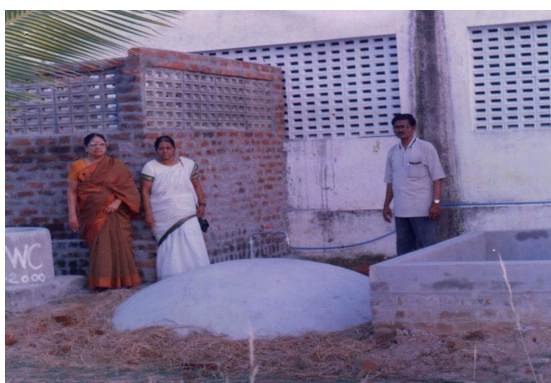
Different rural household biogas plant models in India built by INSEDA. From top left to bottom right: Fixed dome household biogas plant, Grameen Bandhu Model, Deenbandhu Model, KVIC Model.
