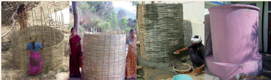
Stages of constructing bamboo reinforced cement mortar water storage tank.
