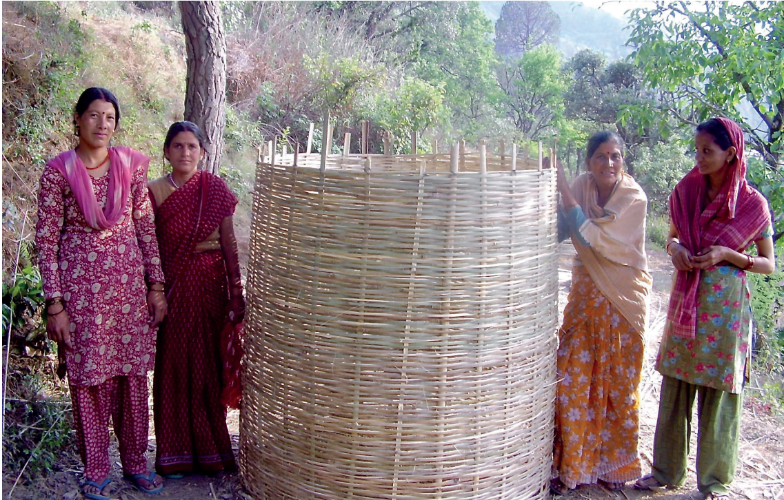
Bamboo reinforcement for rain water tank weaved by these women in India.
