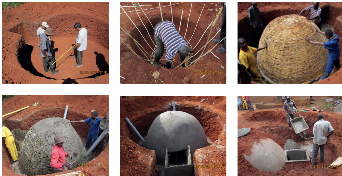
Stages of constructing a household biogas plant.
