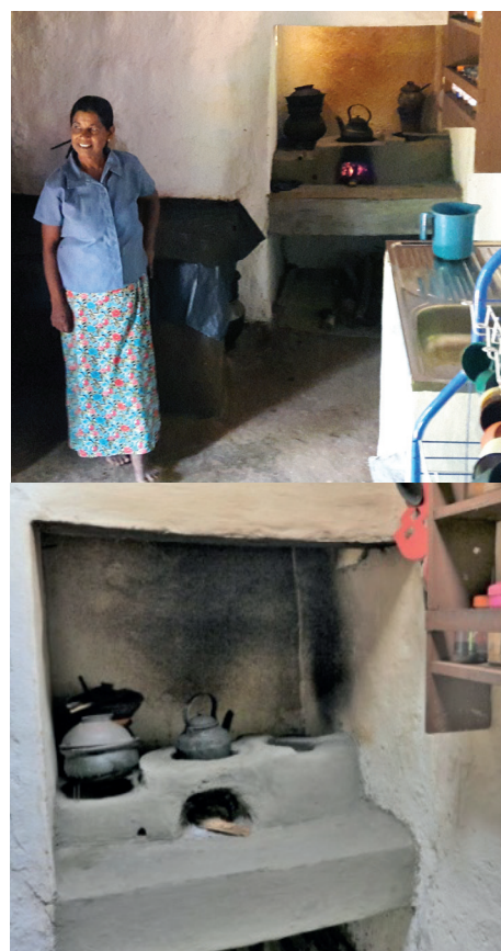
The Anagi stove is typically placed under the chimney hood in the kitchen reducing the smoke in the kitchen.
