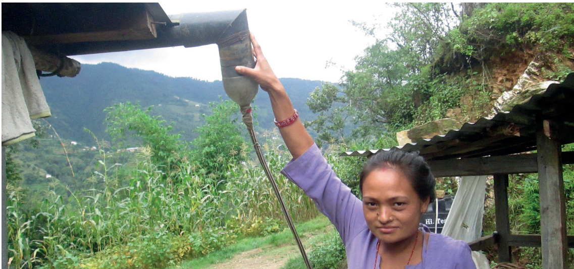
Rain water harvesting set up in the roof of Ms. Rupa's house and a plastic tank to collect water, Chalal Ganesthan VDC.
